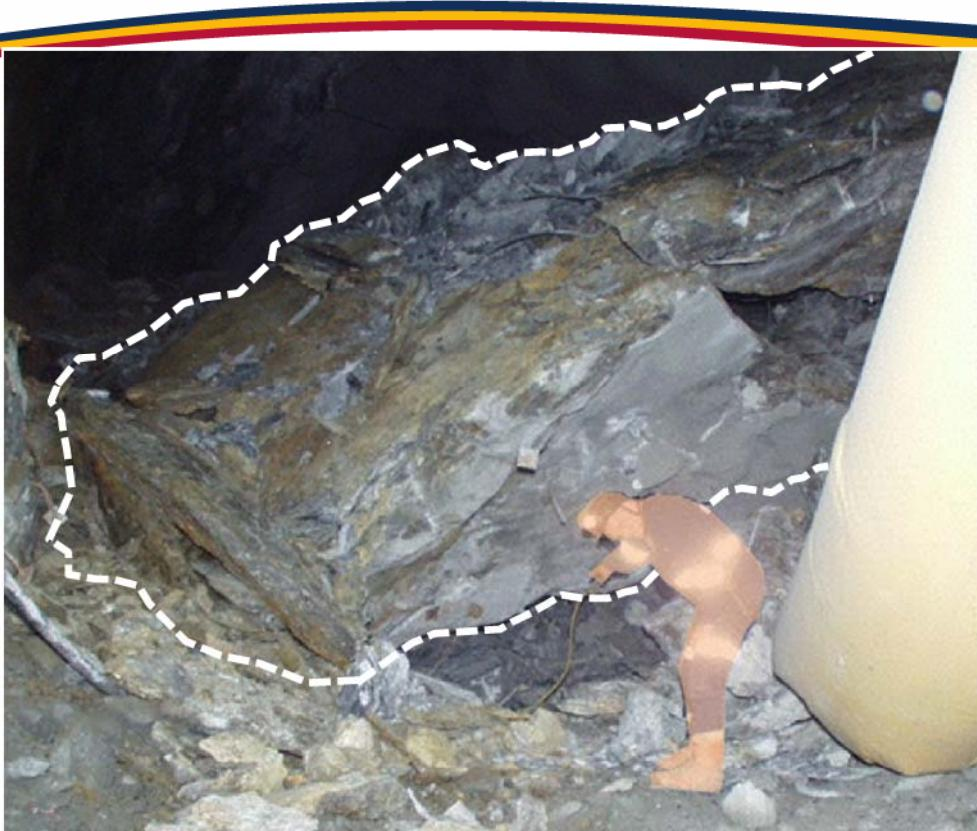
Significant roof failure in a metalliferous mine
