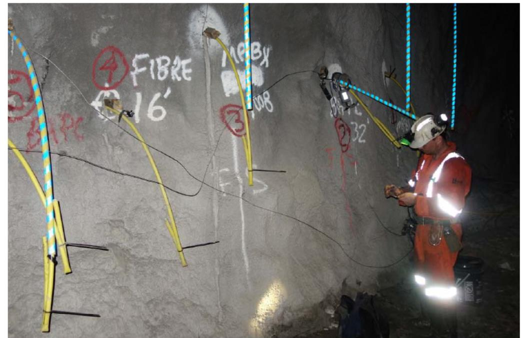
Optical fiber sensors installed at 2.4km depth
